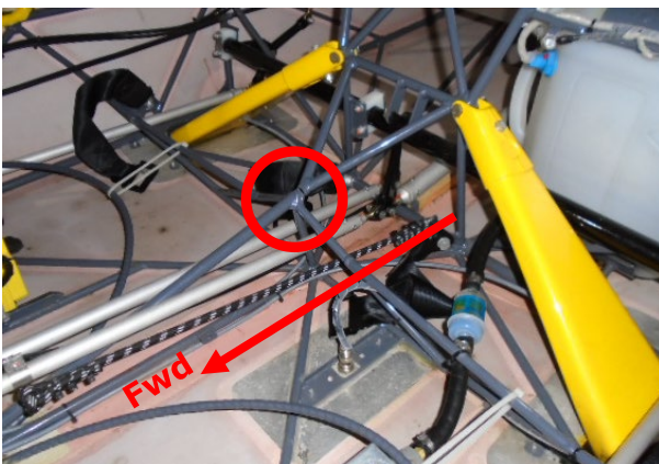
Location of failed weld cluster under seat pan.
