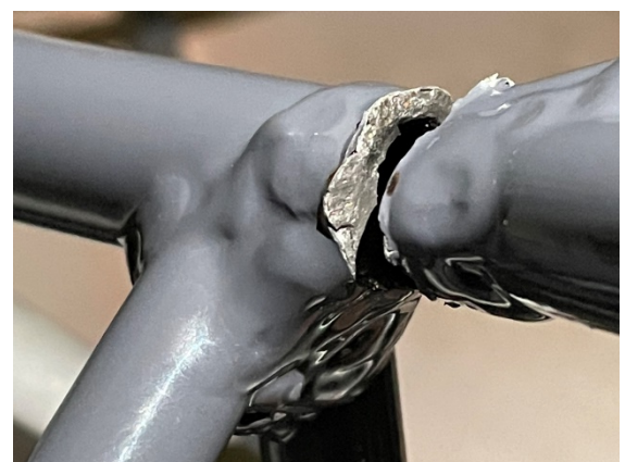
Fracture face of failed weld cluster found located under the seat pan. We have been unable to determine the failure mode due to the apparent burnishing of the fracture surface.
