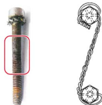
Fig 3 (Left) Shows severe corrosion in a cap-bolt as removed from a Pioneer aircraft operating in a coastal environment, overseas.
