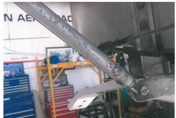
Fig. 3 This picture shows the 'original design' tailplane strut and end fitting – note the corrosion on the strut which should be considered unacceptable.
