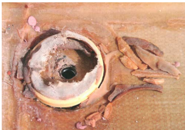
Fig 3. This picture shows an example of a failed fuel strainer. Note that the fine plastic gauze has disintegrated, most likely because of alcohol, now a normal component of mogas.
